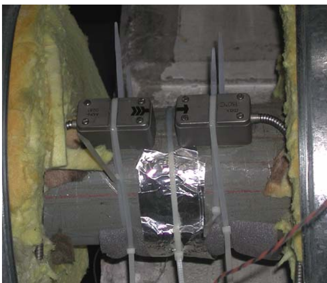
Ultraschall – Flow – Sensor
